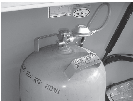
Fig. 110: Gas bottle with pressure reducing valve
