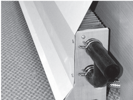
Fig. 87: Convector with thermally conductive panel
